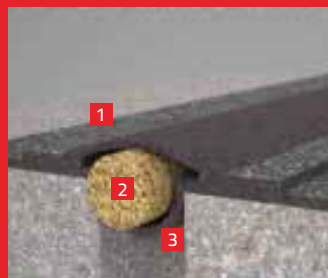
1. Waterproofing layer / 2. PE profile / 3. Flexibit expansion joint
