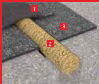
1. Waterproofing layer / 2. PE profile / 3. Flexibit expansion joint
