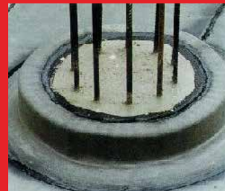
Detail at pile, Flexibit homogeneous bituminous membrane.
